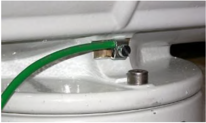
Figure 1-7: Ground Wire Removed
