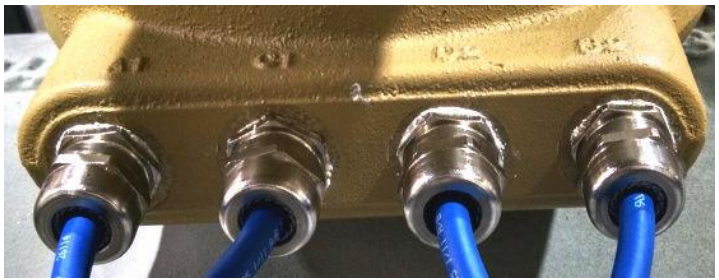
Figure 2-7: Base Enclosure Cable Glands Installation
