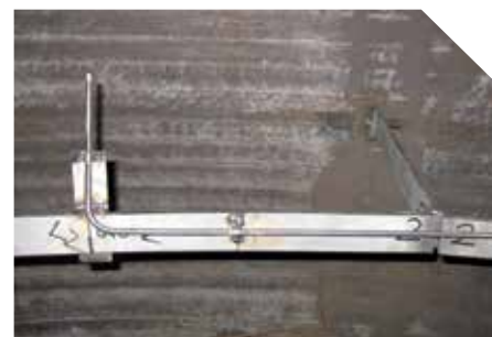
SENSOR ROUTING WITH WELD CLIPS
